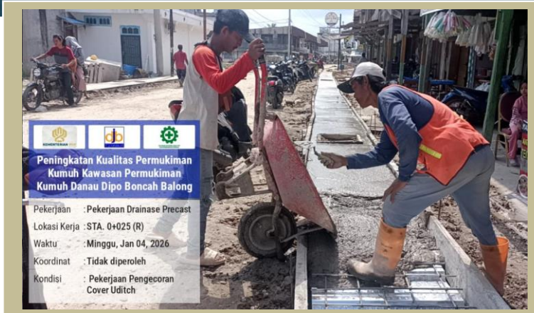
Pek. Pengecoran Cover U-Ditch STA 0+025(R)
