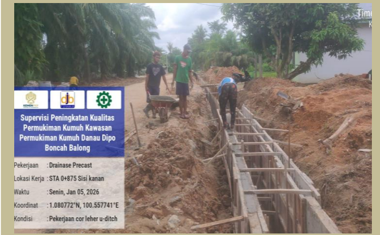
Pek. Pengecoran Leher U-Ditch STA 0+875 (R)
