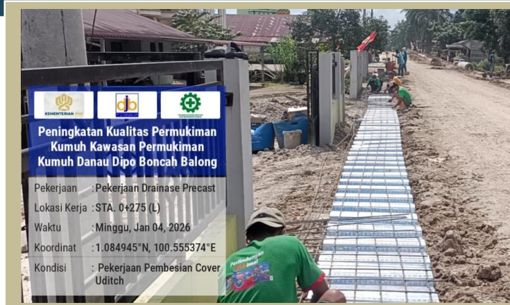
Pek. Pembesian Cover U-Ditch STA 0+175 (L)
