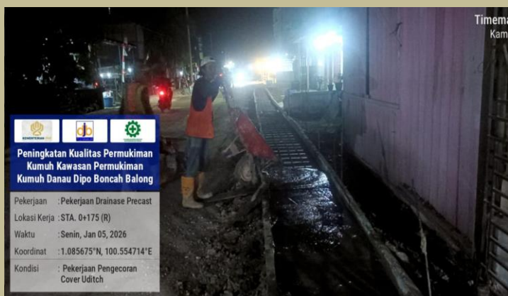
Pek. Pengecoran Cover U-Ditch STA 0+175 (R)
