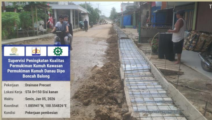
Pek. Pembesian Cover U-Ditch STA 0+150 (R)
