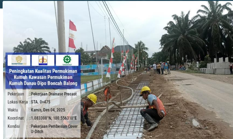
Pekerjaan Pembesian Cover U Ditch STA 0+475
