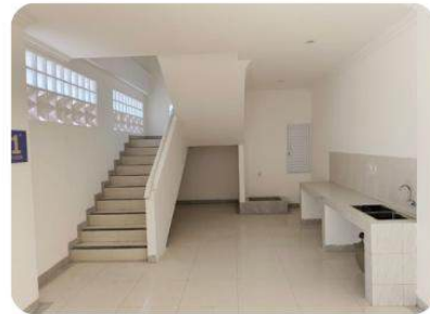
Area Tangga Lantai 1 Wing Kiri
