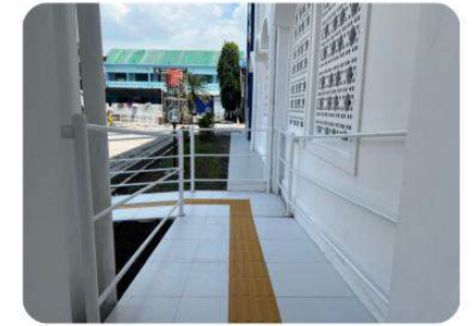
Ramp Difabel Entrance
